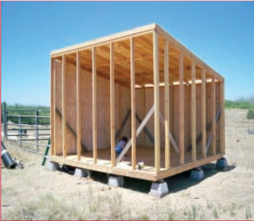
Chicken coop in progress
